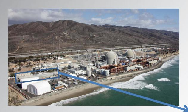
The existing ISFSI storage facility must be increased to accommodate approximately 100 additional canisters
