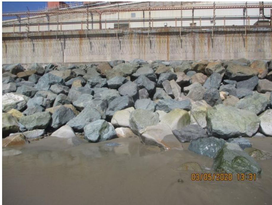
Photo D-18. Photograph taken on 5 March 2020, showing range 18 with a high volume of rocks and minimal beach width along revetment.
