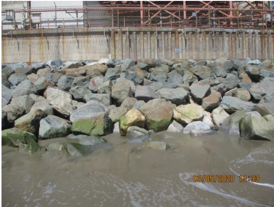
Photo D-19. Photograph taken on 5 March 2020, showing range 19 with a high volume of rocks and minimal beach width along revetment.
