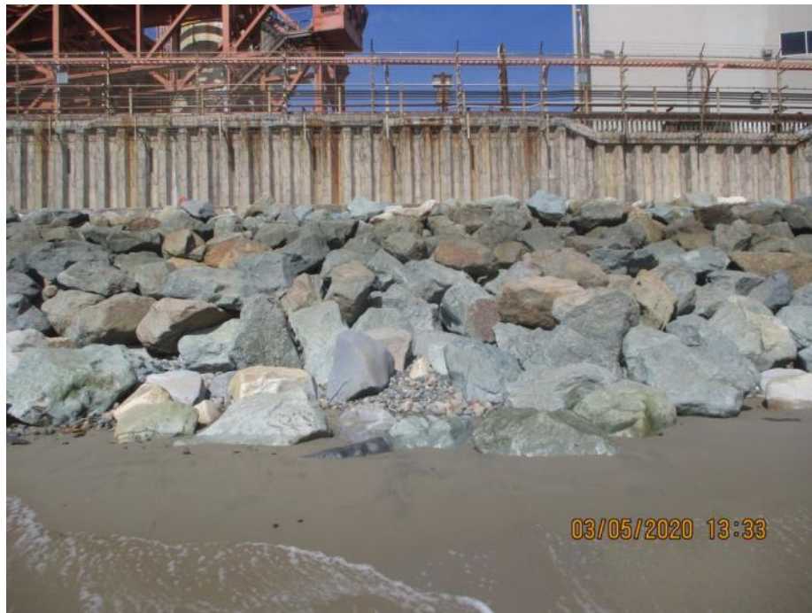
Photo D-20. Photograph taken on 5 March 2020, showing range 20 with a high volume of rocks and minimal beach width along revetment.
