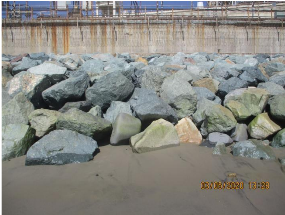
Photo D-17. Photograph taken on 5 March 2020, showing range 17 with a high volume of rocks and minimal beach width along revetment.
