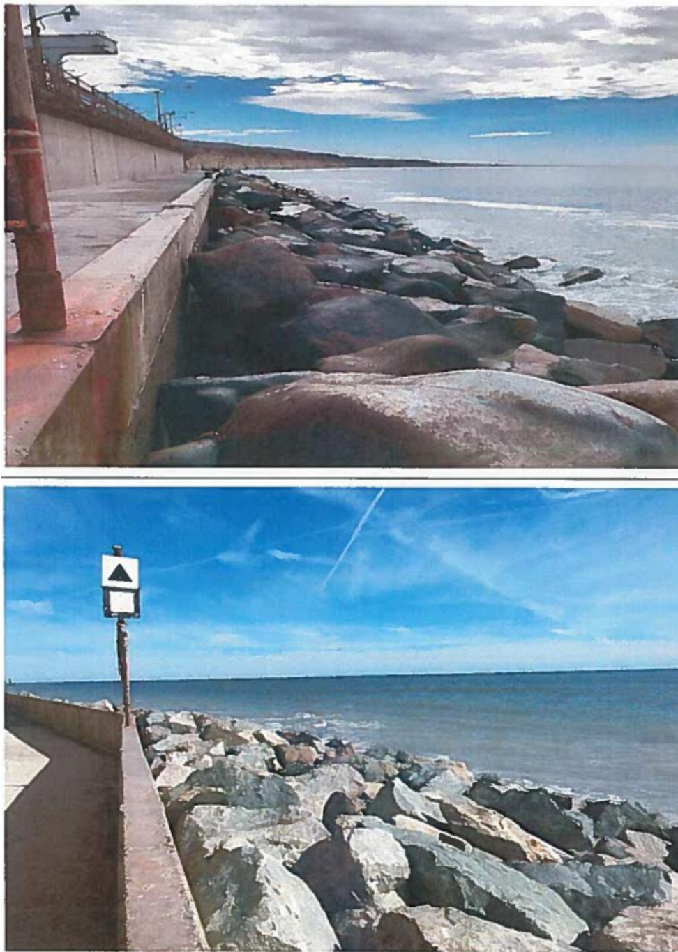
Figure 3-3. Top photograph taken on 20 March 2018, before placement of riprap. Bottom photograph taken on 17 December 2019, after placement of riprap within gaps and depredated areas of the revetment. Direction of the photograph taken towards the south.
