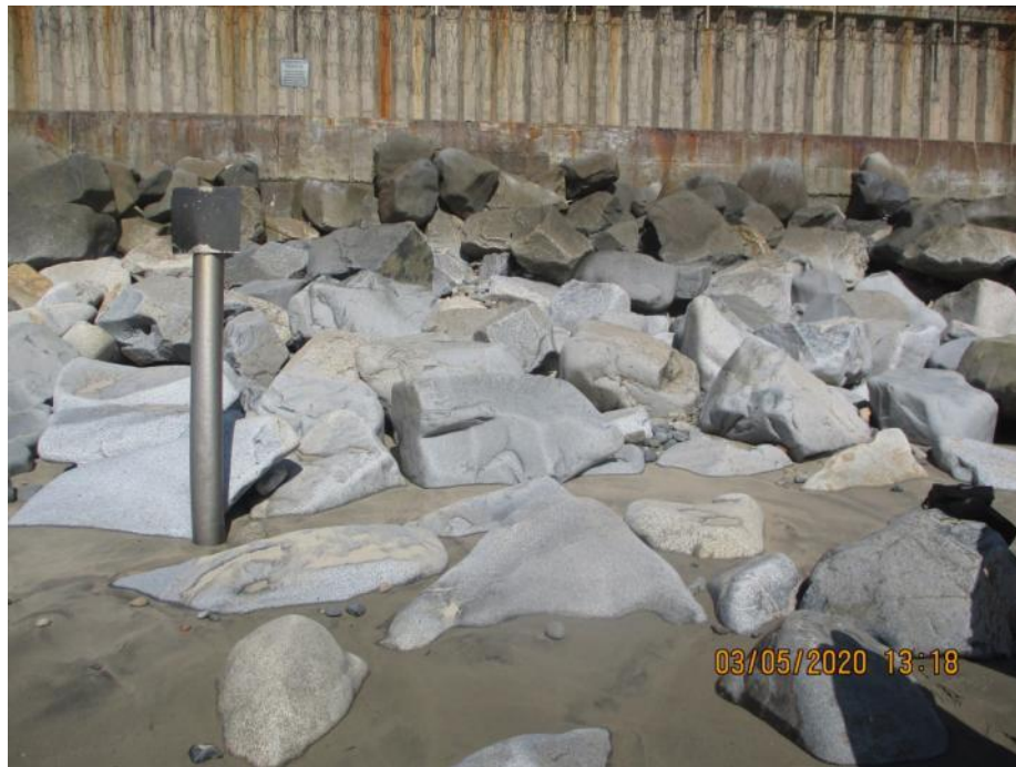
Photo D-14. Photograph taken on 5 March 2020, showing range 14. Seaward base of revetment partially covered with sand.
