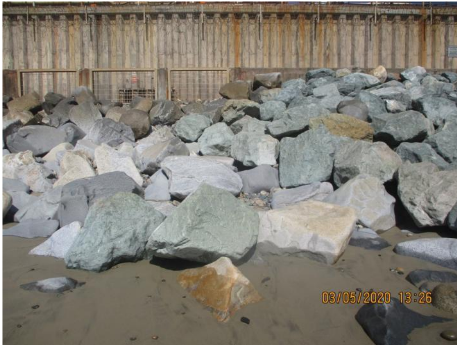
Photo D-15. Photograph taken on 5 March 2020, showing range 15 increasing in revetment volume with decreasing beach width.
