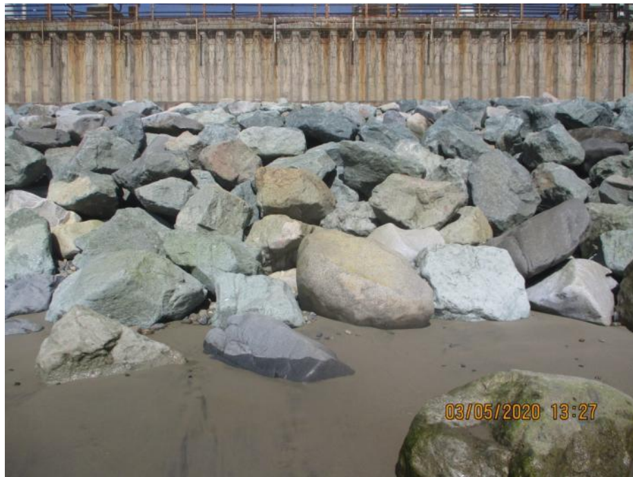
Photo D-16. Photograph taken on 5 March 2020, showing range 16 with a high volume of rocks and minimal beach width along revetment.
