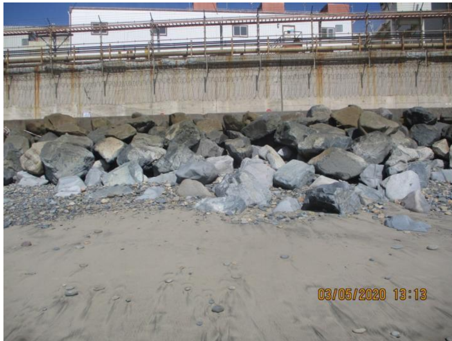
Photo D-12. Photograph taken on 5 March 2020, showing range 12 partially covered with sand and cobbles.
