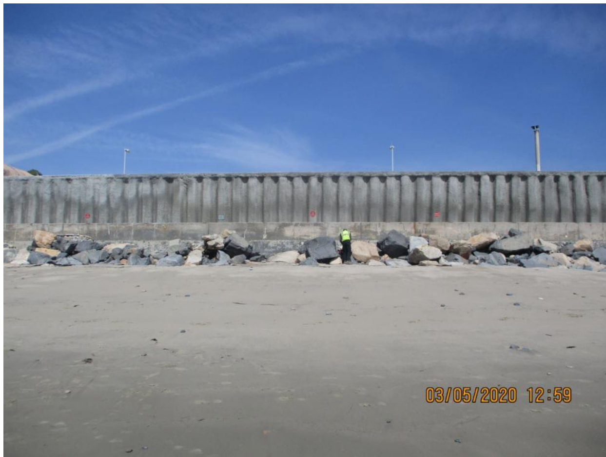
Figure 3-19. North portion of the revetment covered by beach sand.
