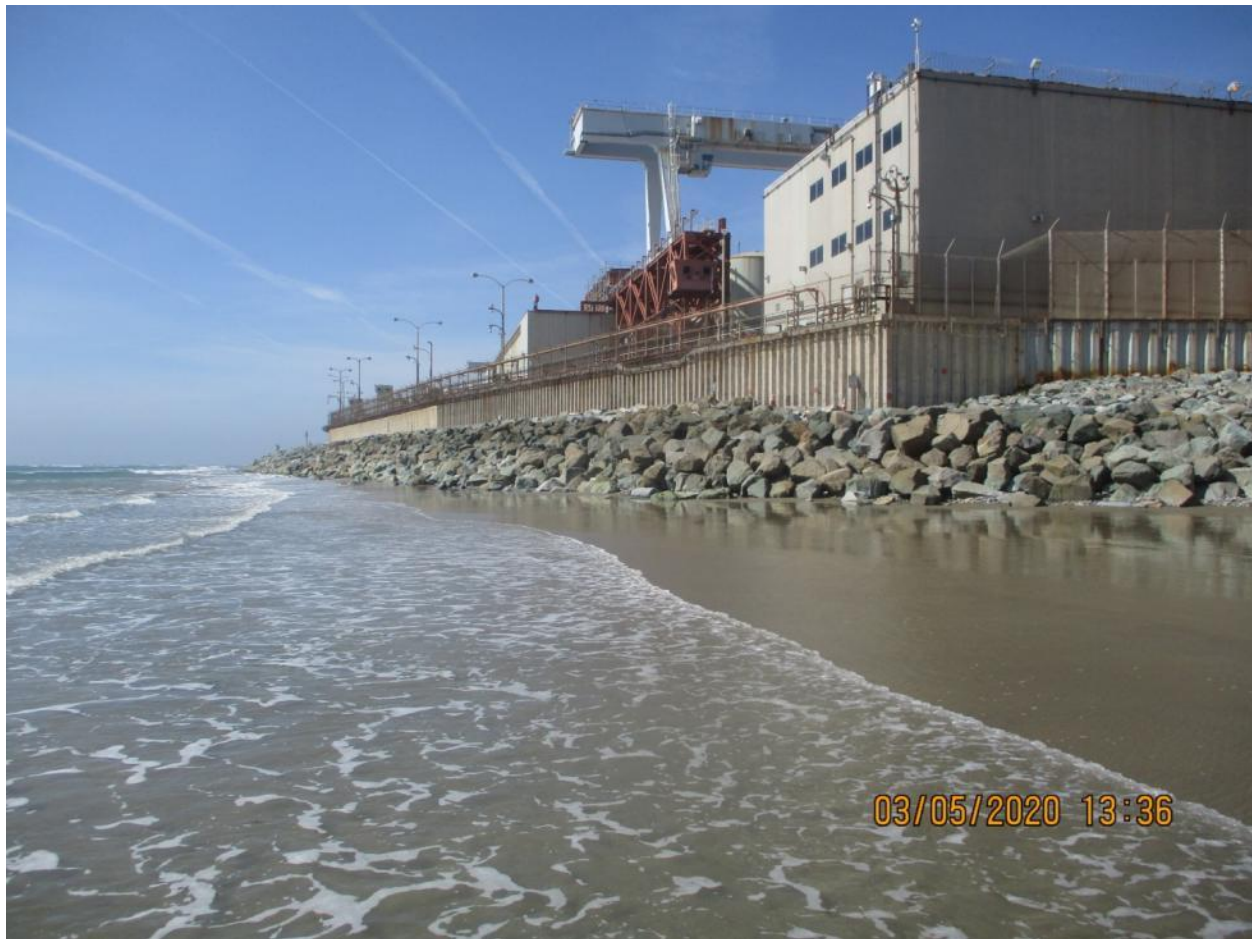
Figure 3-2. Close up of the revetment at its southern end.
