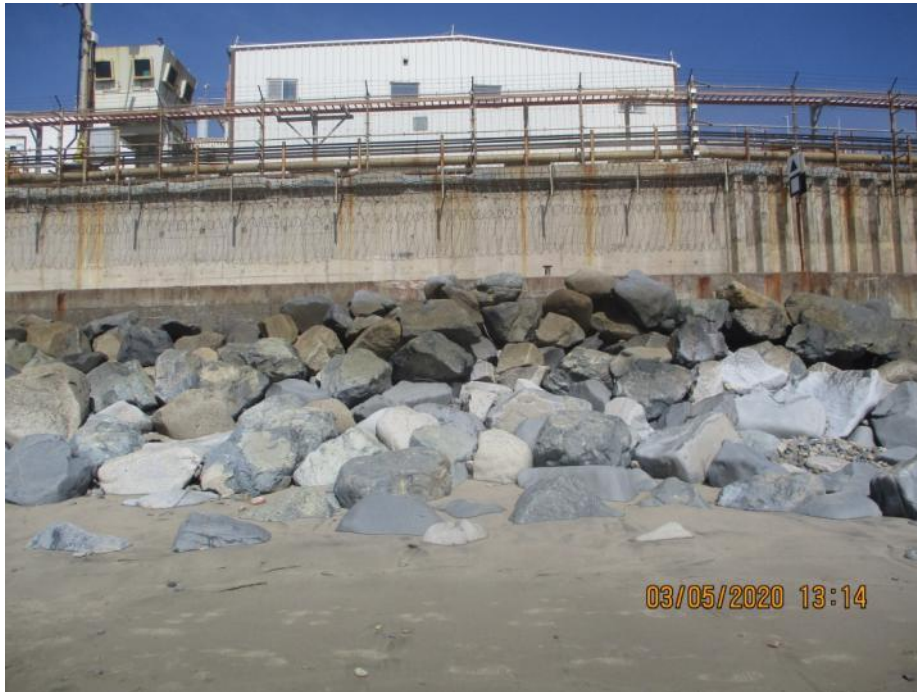
Photo D-13. Photograph taken on 5 March 2020, showing range 13. Seaward base of revetment partially covered with sand.
