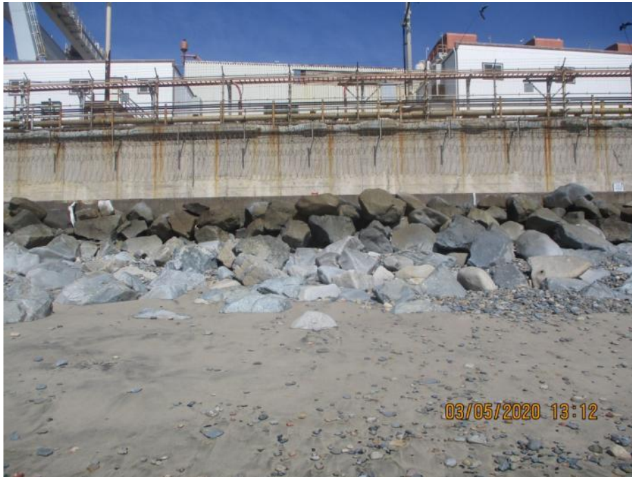
Photo D-11. Photograph taken on 5 March 2020, showing range 11 partially covered with sand and cobbles.
