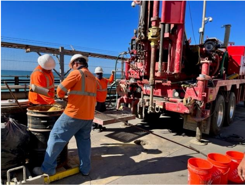
Photo 1 –Using mobile drill rig to collect soil samples for testing (February 17, 2022).
