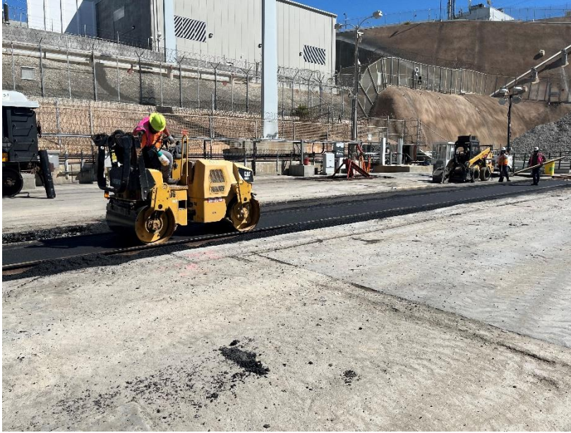
Photo 5 – Asphalt application at rail tracks (February 28, 2022).
