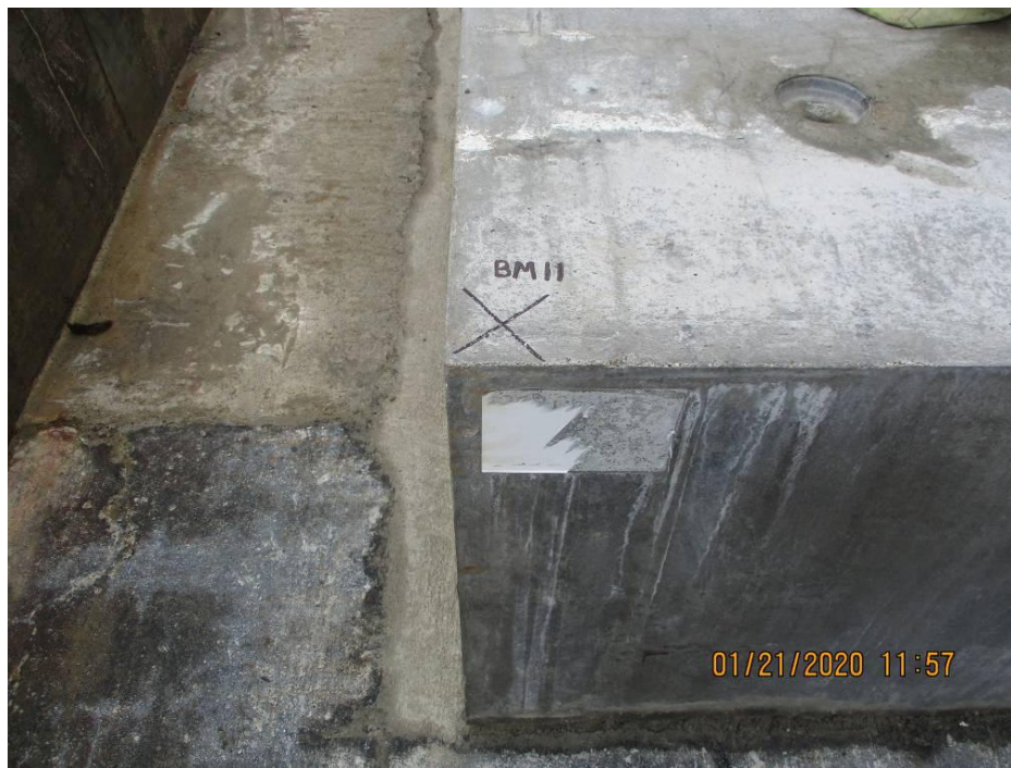
Photo B-21. Benchmark BM11, created on 21 January 2020, is located on top of the concrete blocks at the southern end of the SONGS walkway.
