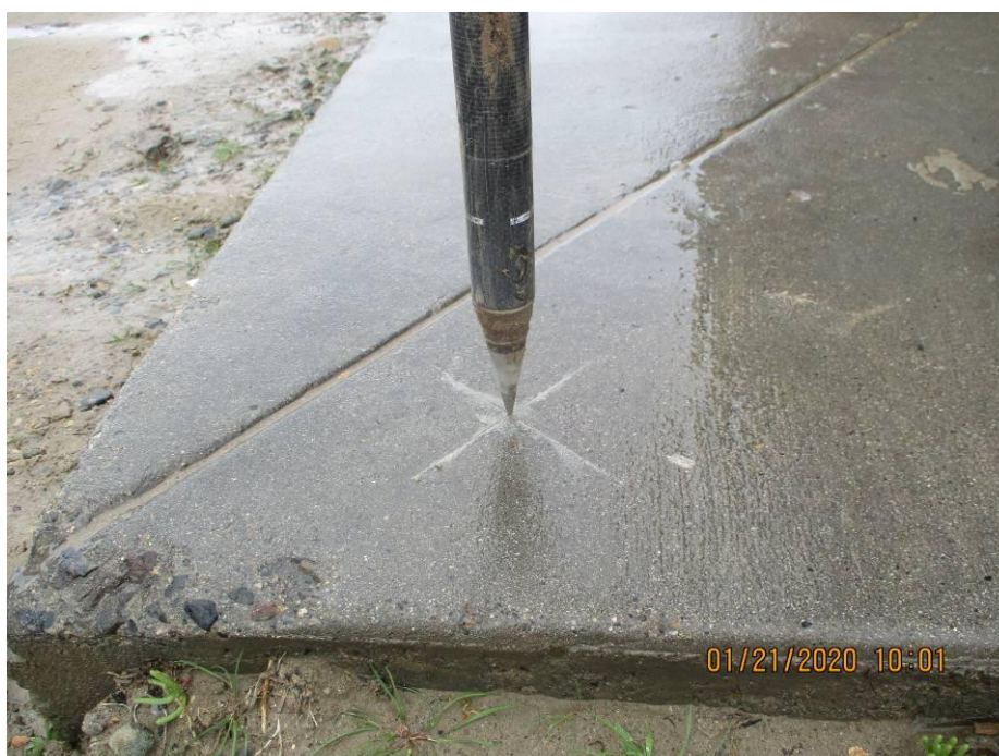
Photo B-16. Benchmark BM02, created on 21 January 2020, is located on the SW corner of Bathroom 2 in the San Onofre State Beach parking lot. Benchmarks BM02 through BM06 are all marked by a scribed X on the concrete foundation.
