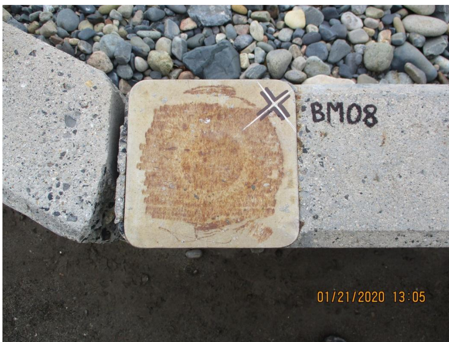
Photo B-18. Benchmark BM08, created on 21 January 2020, is marked by a scribed X and located just south of transect NS0000 on top of the seawall.
