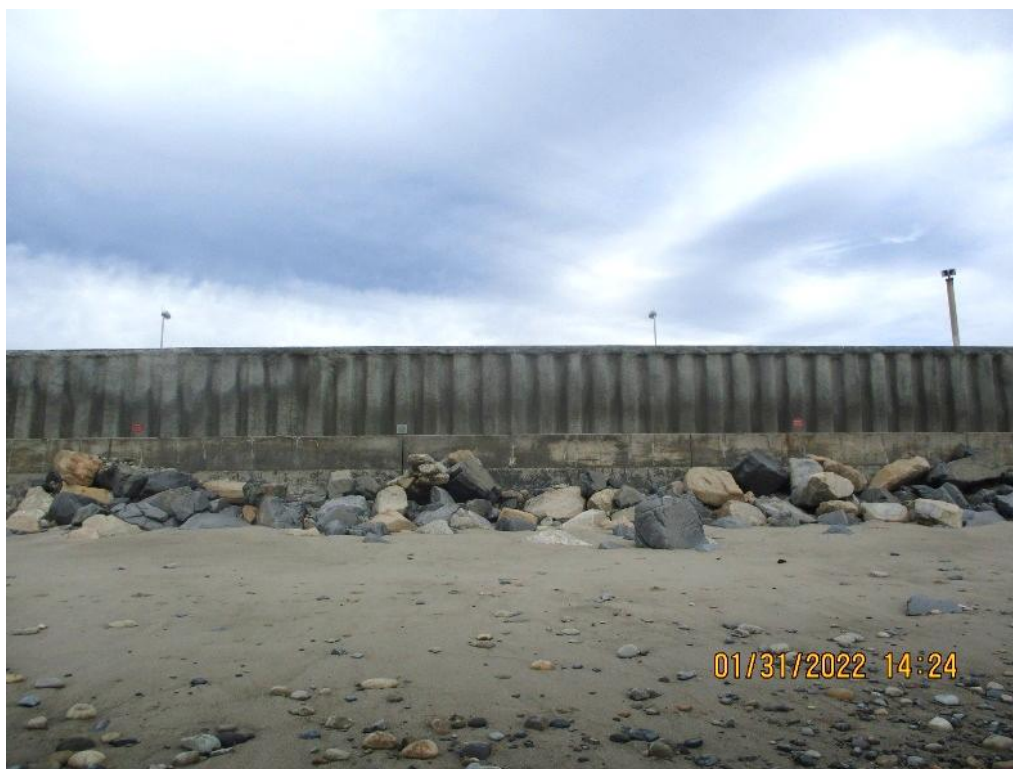
Figure 3-24. North portion of the revetment (Range 3) covered by beach sand in 2020 (top), and a small amount of cobbles exposed in 2022.
