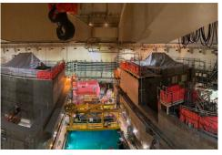
Inside Unit 3 containment - the removal and cutting of main components such as the reactor coolant pumps, reactor vessel were completed in 2023.
