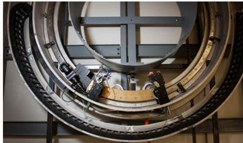
AREVA inspection ring
